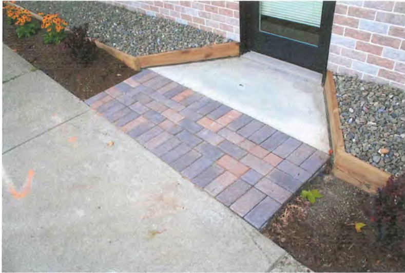
Proposed brick pavers to extend sidewalk at Meadow St & Seneca Street Corner
