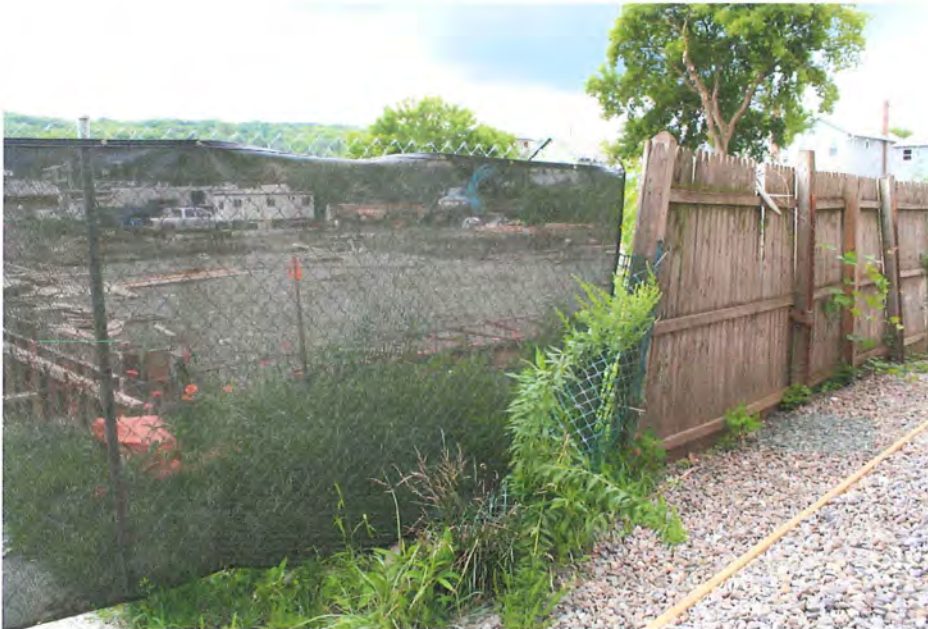
Planned Parenthood construction pit, which runs to property boundary.
