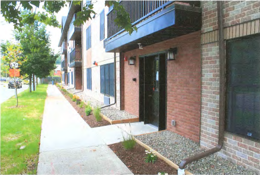
Old fashioned “lamp” style fixtures at the building entrances.
