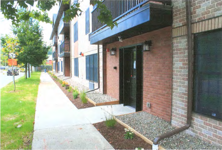
A Landscaping strip was planted outside of the foundation extension, and a new street tree was planted along Seneca Street.
