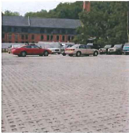
Clipper Mill, Baltimore, MD; Owner/Developer: Struever Bros, Eccles & Reuse; Size & Color: EcoGrid®, Natural; Finish: Natural
